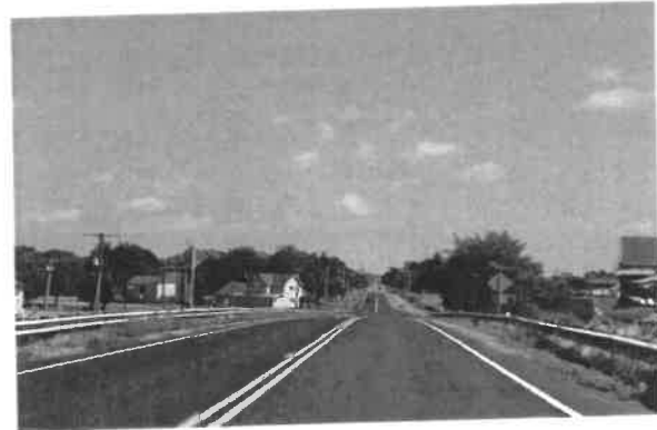
County Road 313 - After Resurfacing
