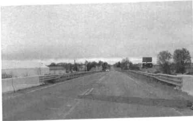
County Road 313 - Prior to Resurfacing
